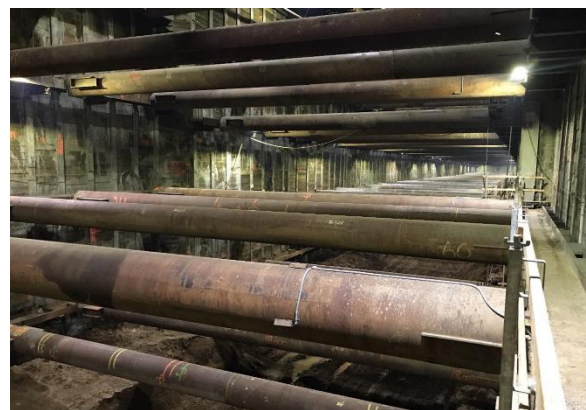
Wilshire/Rodeo Station Excavation Support
