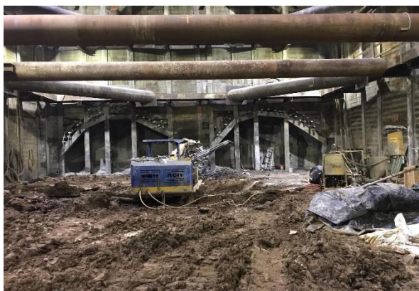
Canopy Pipe Drilling Wilshire/Rodeo Station
