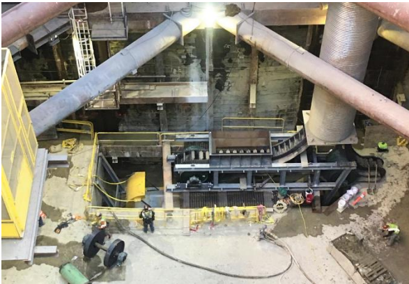
Preparation for Tunneling Transition to Tunnel Access Shaft (TAS)
