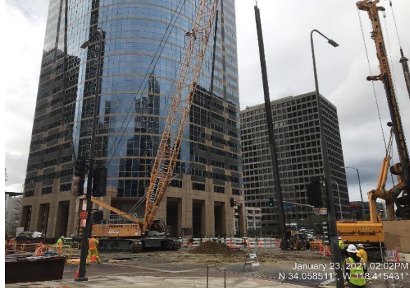
Pile Installation West of the LB in Century City
