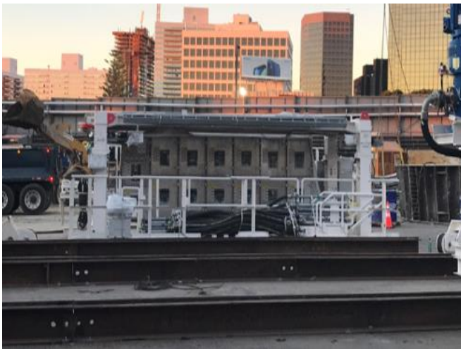
BR TBM Assembly of Trailing Gantries
