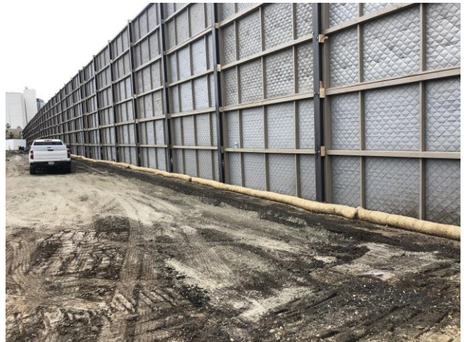
Sound Wall Installation at Westwood/VA Station Site (VA Lot 42)
