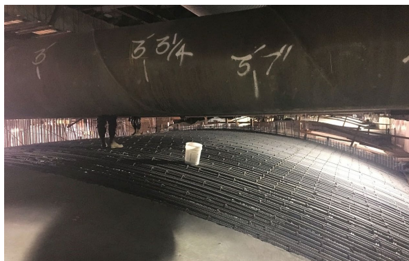
Roof Rebar Placement at Wilshire/Fairfax Station
