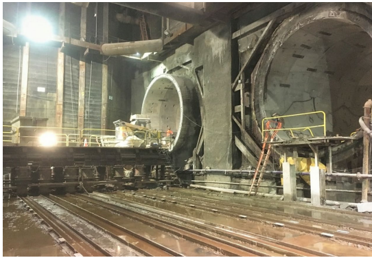
View of Wilshire/Western Shaft
