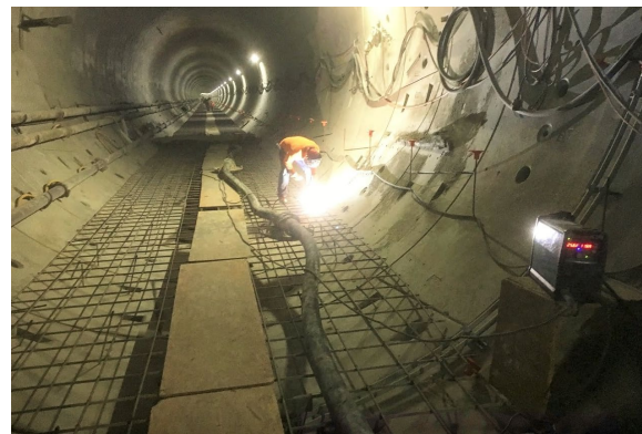
Rebar Placement at Reach 1 Tunnel
