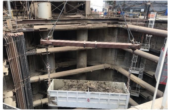
Muck Removal at the Tunnel Access Shaft
