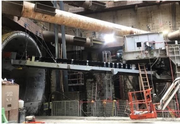
Muck Removal at the Tunnel Access Shaft
