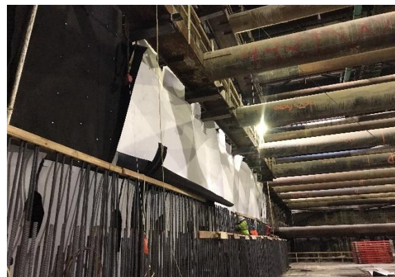
Wilshire/Rodeo Station Waterproofing Membrane, Rebar and Formwork for First Level Walls
