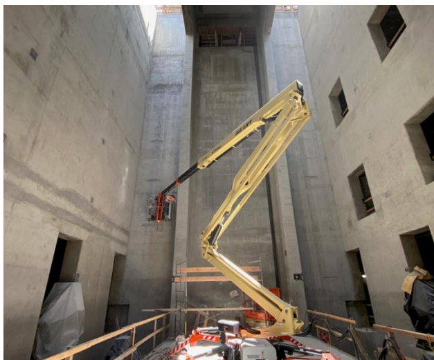
Station interior at Grand Av Arts/Bunker Hill Station
