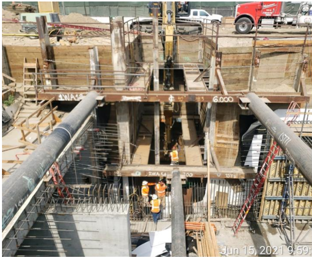
Excavation & SOE at emergency stairs at Alameda/Temple
