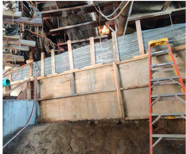
Stripping slurry forms in east Hammerhead at Historic Broadway Station
