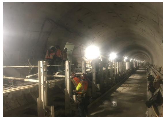
Reach 1 Walkway Formwork Installation
