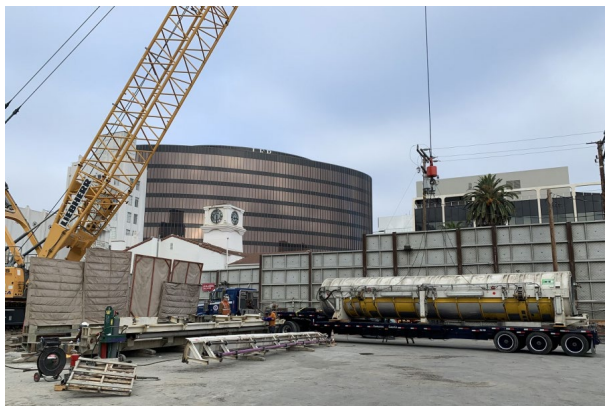
TBM Gantry Components Loaded on Truck
