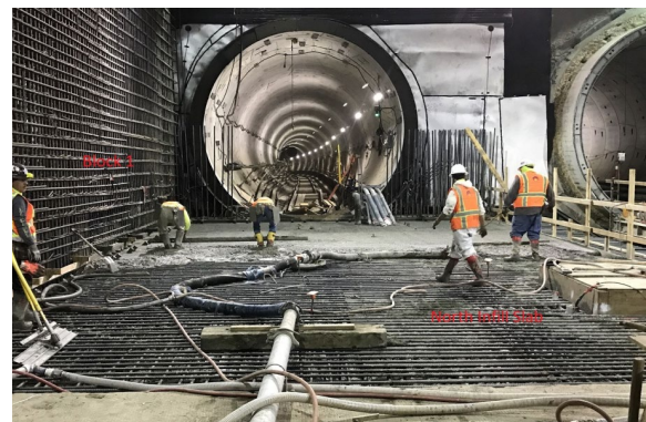
Infill Slab Concrete Work at Wilshire/La Cienega Station
