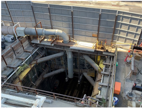
View of Wilshire/Western Shaft
