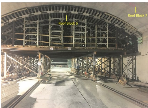
Roof Formwork Assembly at Wilshire/Fairfax Station
