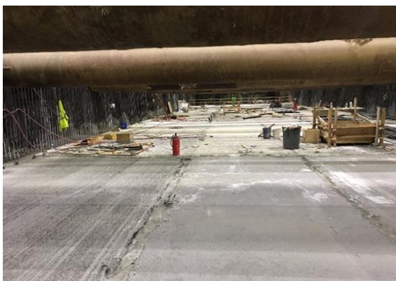
Wilshire/Rodeo Station Invert Slab Preparation
