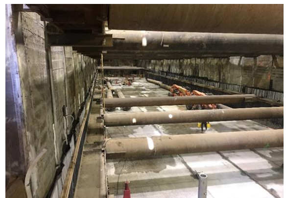
Wilshire/Rodeo Station Invert Slab Preparation
