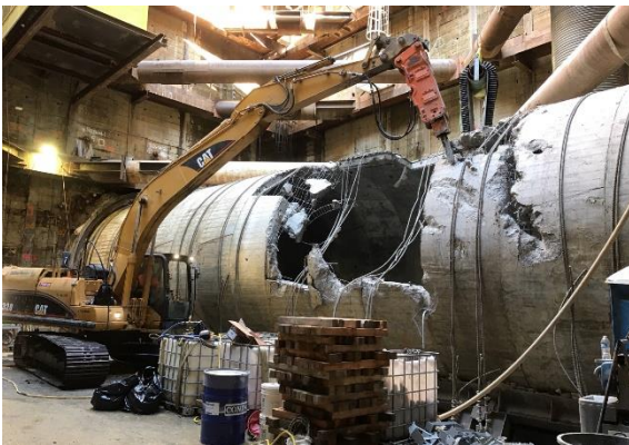
BL Temporary Ring Removal TAS in Century City
