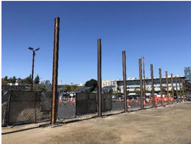
Installation of Noise Barrier Wall Piles at Westwood/VA Station
