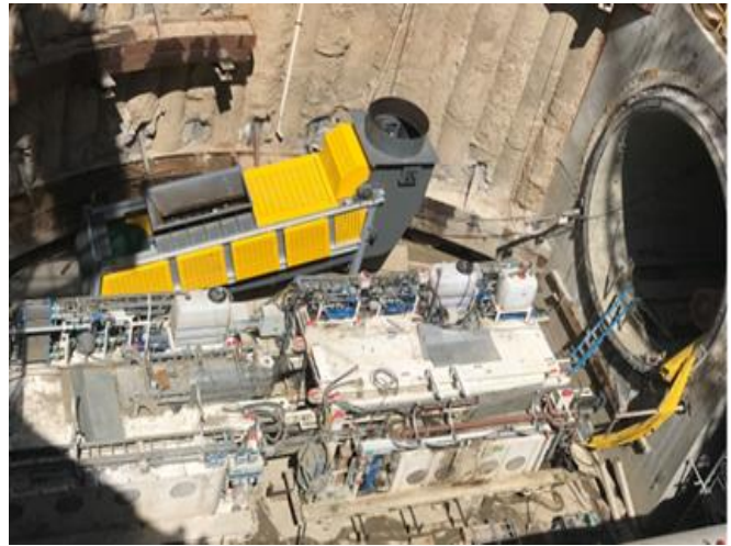
Assembly of Vertical Belt Structure at Tail Track Exit Shaft
