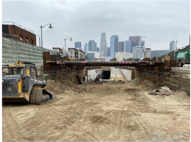
1st St U-Channel – Excavation to Subgrade at 1st Street Leg
