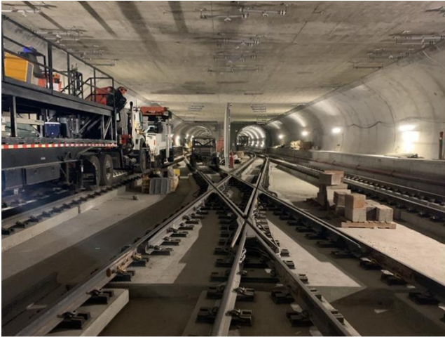
No. 8 Double Crossover adjacent to Historic Broadway Station
