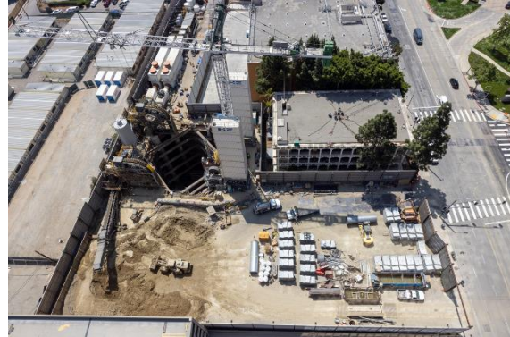
Tunnel Access Shaft in Century City
