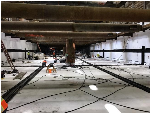
Wilshire/Rodeo Station Invert Slab Preparation
