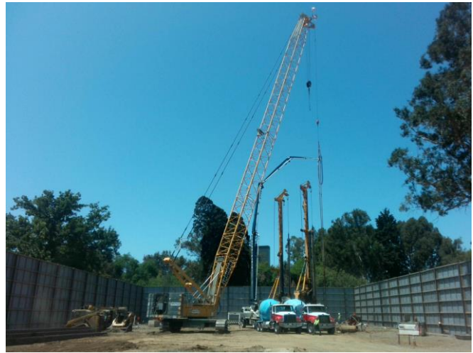
Concrete Pour in Process for Installation of Support of Excavation Soldier Piles at Westwood/VA Station
