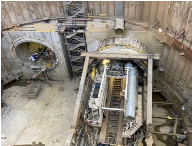
TBM Assembly Overview at Tail Track Exit Shaft
