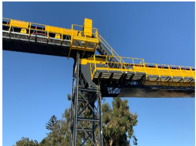
Assembly of Conveyor Belt Walkway at Tail Track Exit Shaft
