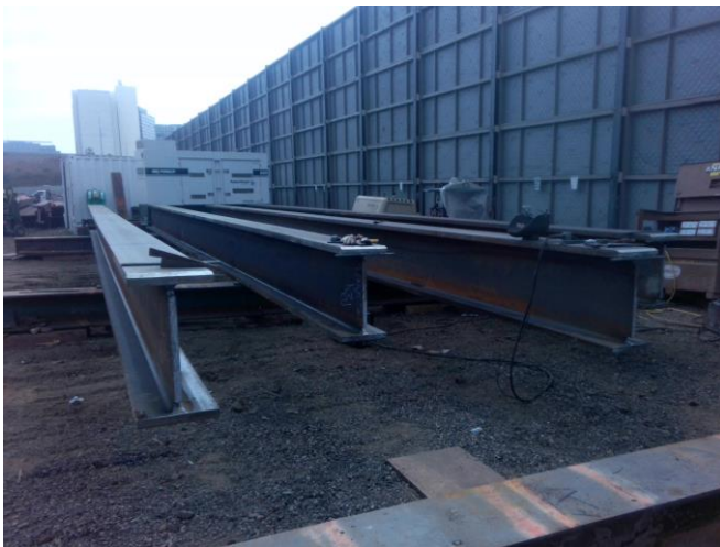
Pile Fit Up at Westwood/VA Station
