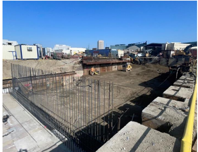
Wye Fan Plant TBM Backfill
