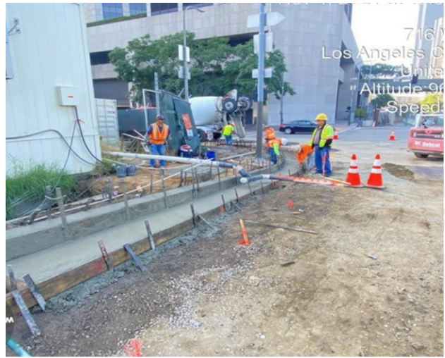
3rd/Flower NE Corner – Curb and Gutter Placement
