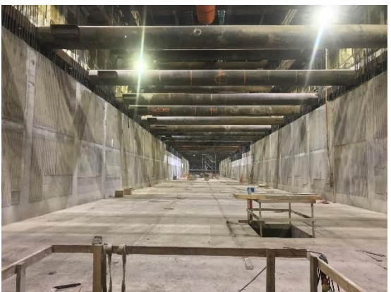
Concrete Placement for First Level Station Walls
