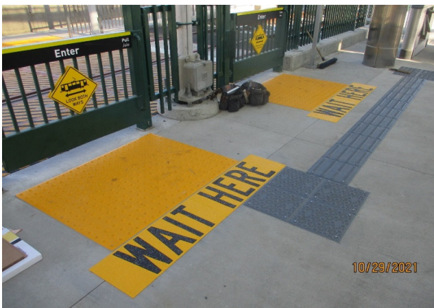
LA BREA STATION – Applying the “Wait Here” stencils at the La Brea Station
