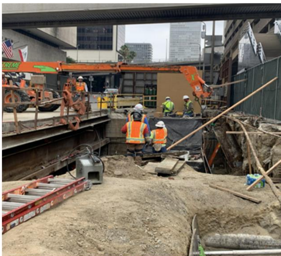
Removing soldier piles on Flower St
