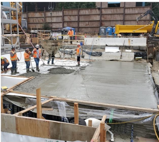
Historic Broadway Station LTS1 slurry backfill
