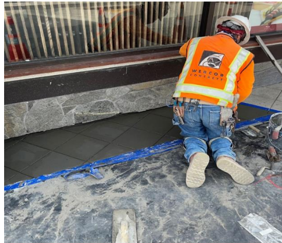
1st/Central decorative paving restoration
