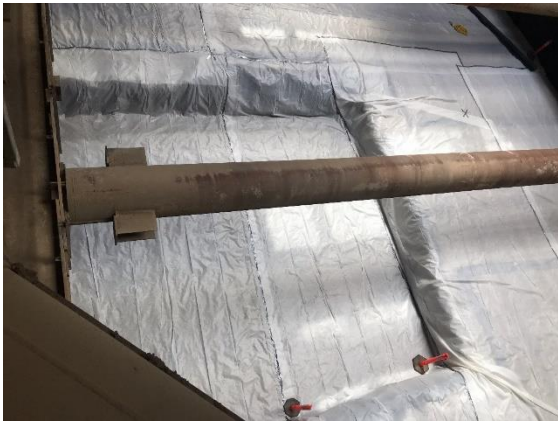
Wilshire/Rodeo Station Waterproofing Membrane, Rebar and Formwork for Station Entrance
