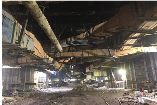
Excavation Activities West of the Launch Box in Century City
