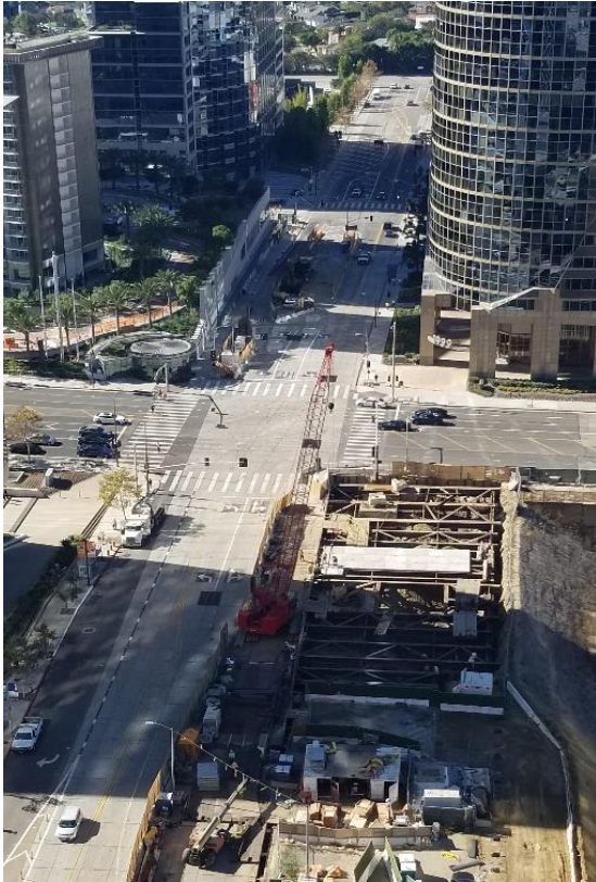
Station Entrance Deck Beam Installation in Century City
