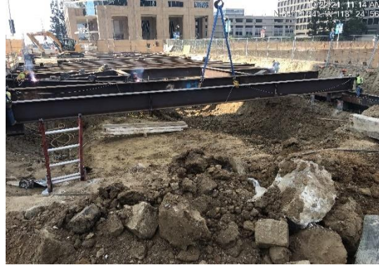
Station Entrance Deck Beam Installation in Century City
