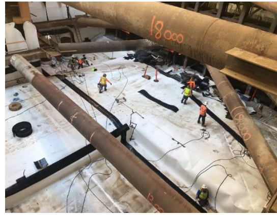
Wilshire/Rodeo Station Waterproofing Membrane, Rebar and Formwork for Station Entrance
