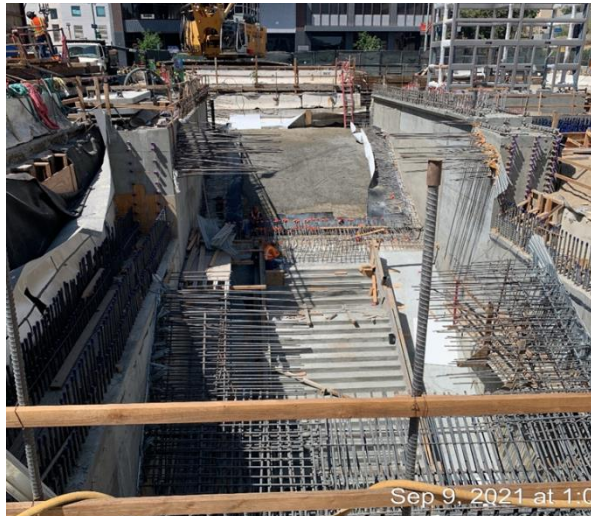
Historic Broadway Station Entrance Structure Roof
