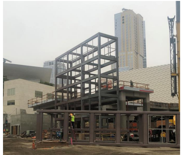
Grand Av Art/Bunker Hill Station Entrance Structure and Ped Bridge
