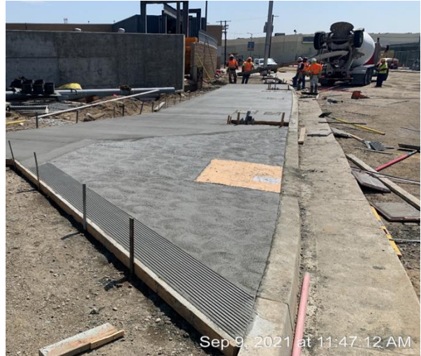
Temple Street Restoration – North Ramp/Sidewalk Pour
