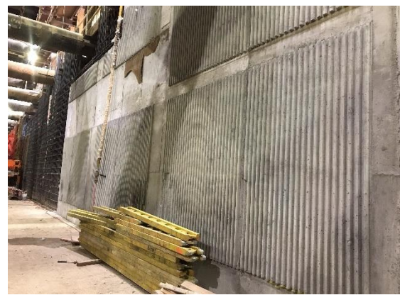
Concrete Placement for First Level Station Walls
