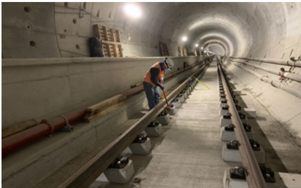
Reach 1 (South) Track Installation
