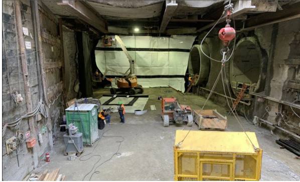
Waterproof Membrane Installation at Wilshire/Western Shaft
