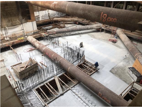
Concrete Placement at Wilshire/Rodeo Station Entrance for Invert Slab
