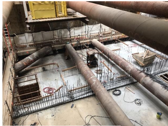
Concrete Placement at Wilshire/Rodeo Station Entrance for Invert Slab
