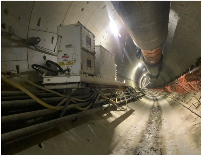
BL Tunnel Booster Fan & Transformer Installation In Progress
