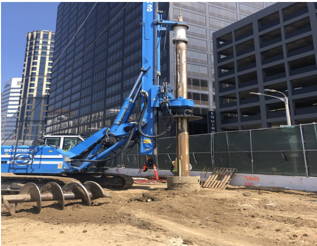
Westwood/UCLA Station Dewatering Well Drilling in Progress
