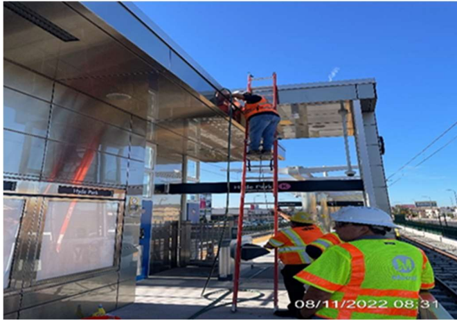
Hyde Park Station - WSCC preparing to conduct water leak test
