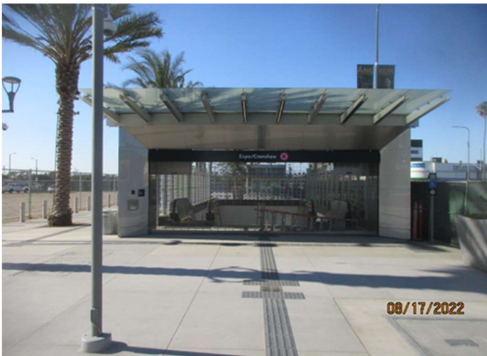
Expo Station - main entrance at the plaza.
