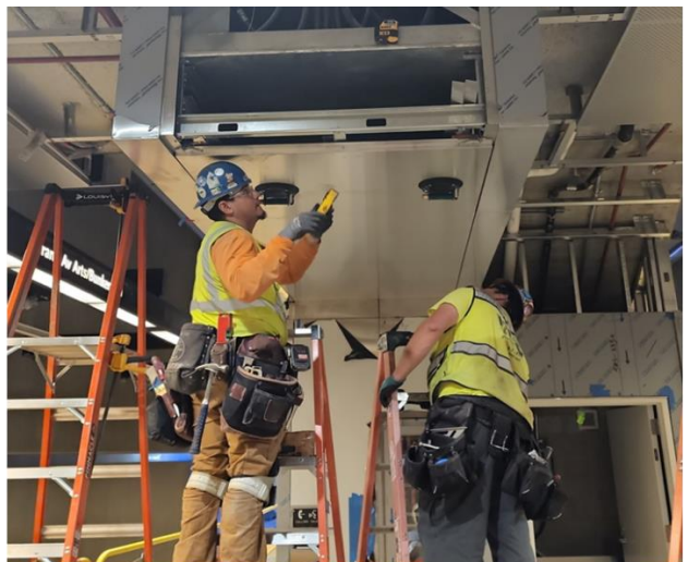
Platform – Stainless Steel Cladding Installation at Grand Av Arts/Bunker Hill Station
