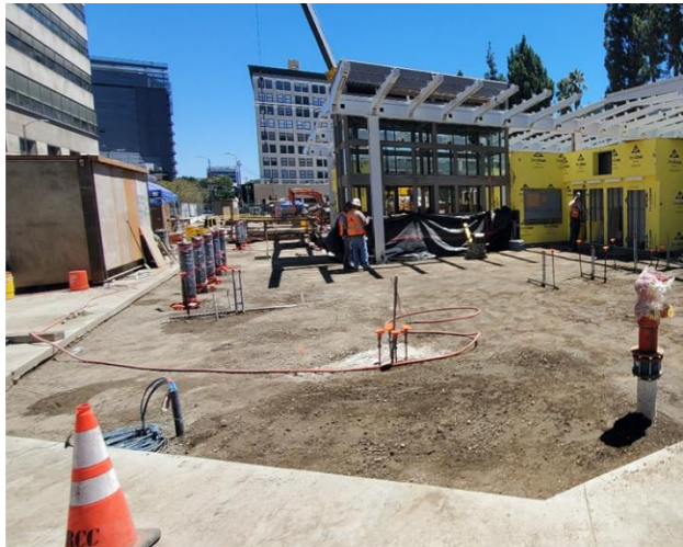
Concrete placement for entrance level at Historic Broadway Station
