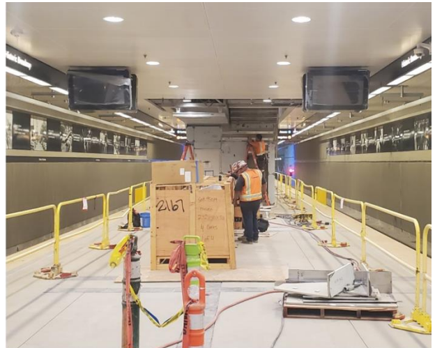
Platform level at Historic Broadway Station
