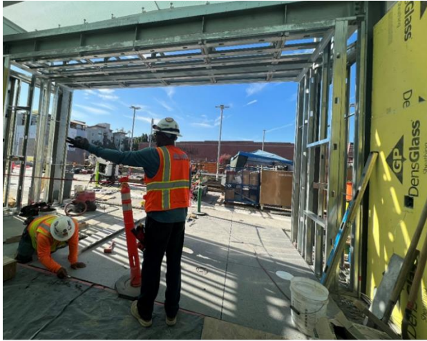
Granite tile placement at elevator area at Little Tokyo/Arts District Station
