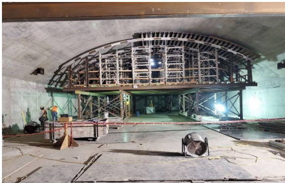
Removing Roof Falsework at Wilshire/Fairfax Station
