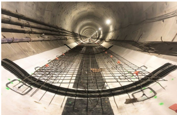
Reach 2 Invert Rebar
