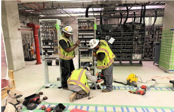
Installing Equipment Racks at Wilshire/Western
