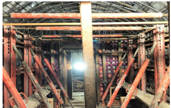
Reach 3 Cross Passage #22
