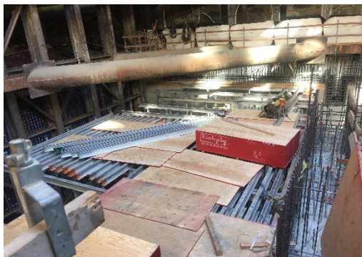
Station Entrance Concourse Level Roof Slab Rebar Installation at the Wilshire/Rodeo Station
