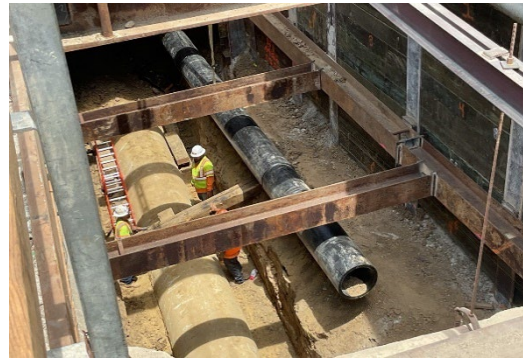
Sewer Bypass and Storm Drain Realignment Activities in Century City
