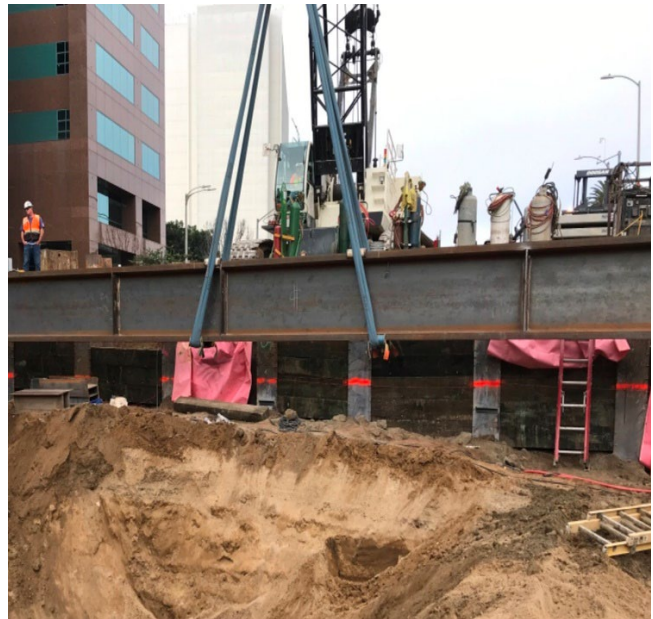
UCLA Station: Installing Structural Steel Beams for Temporary Decking
