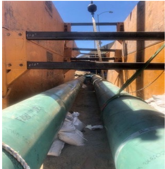
Steam Tunnel Redundant Line: Installed & Connected 6" & 10" Prema Pipe Weld Joints
