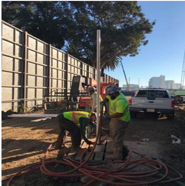
Install Geotechnical Instrumentation at VA
