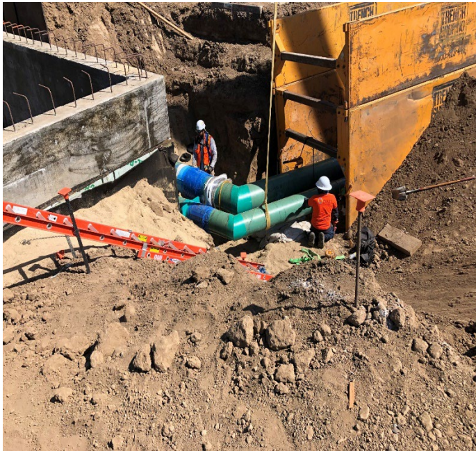
VA Steam Tunnel: Installing Redundant System (Condensate and Steam Line)
