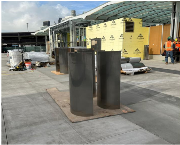
Stainless steel cladding delivery at Little Tokyo/Arts District Station
