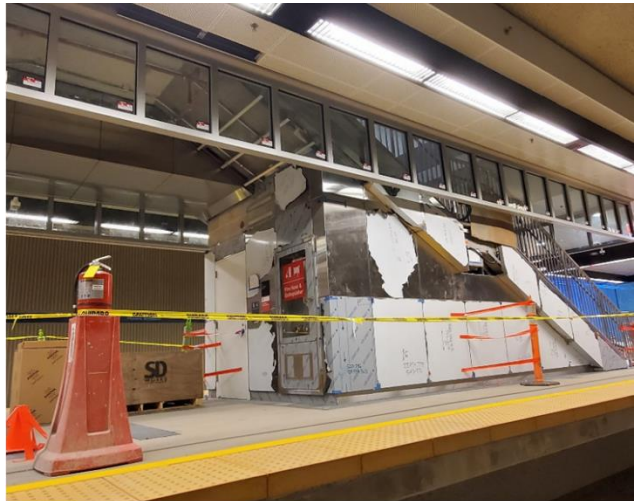
Installation of stainless-steel cladding around stairs at Historic Broadway Station
