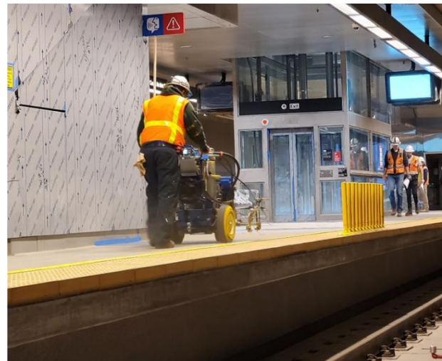
Platform level painting at Grand Av Arts/Bunker Hill Station
