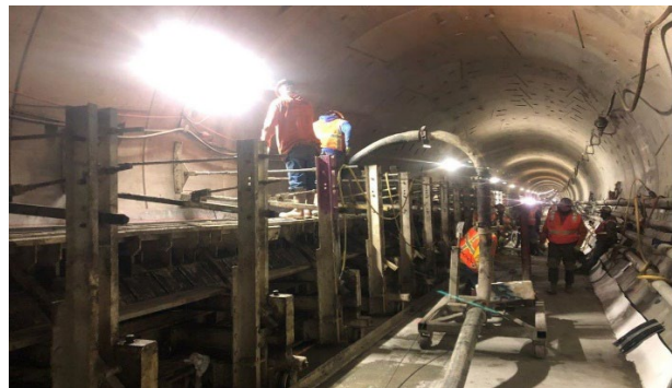
Reach 3 BL Tunnel Walkway Construction
