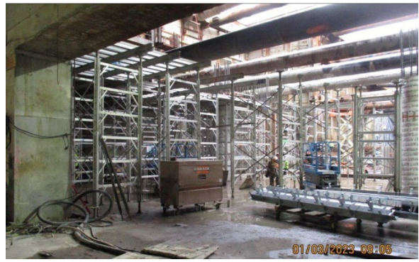
Wilshire/La Brea Station Entrance Structure Roof Shoring
