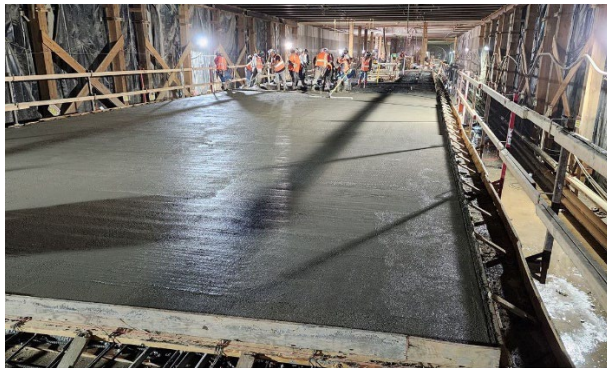
Wilshire/Fairfax Station Platform Construction
