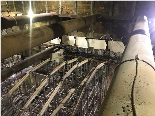
Concourse Level Roof form Work at the Wilshire/Rodeo Station Box
