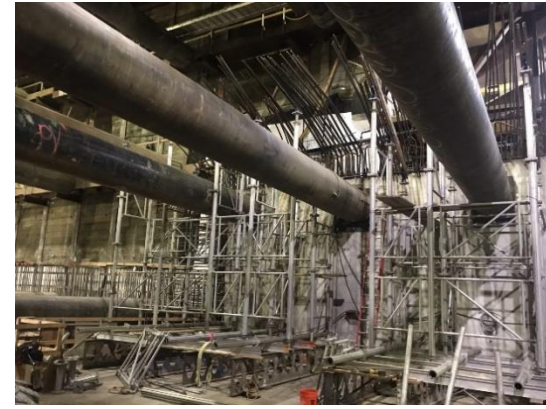
Concourse Level Roof form Work at the Wilshire/Rodeo Station Box
