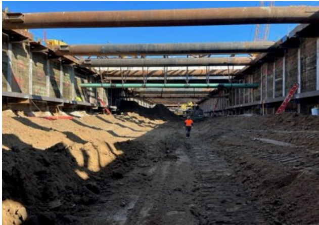
Westwood/VA Station – Installation of Struts & Strain Gauges; Sanitary Sewer Lines Supported
