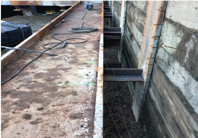
Westwood/UCLA Station – Waler (EW-6) Placement on West Side of Main Entrance
