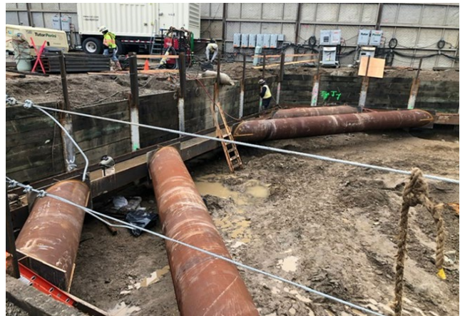
Westwood/UCLA Station – Installation of Lagging, Wale Supports, and Corner Braces
