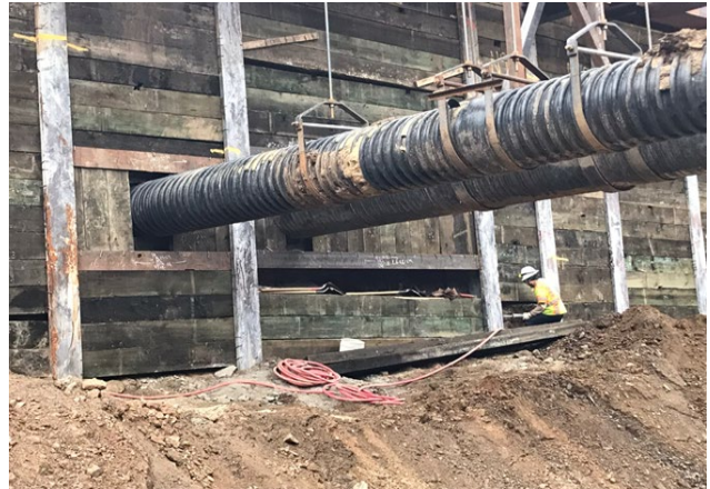
Westwood/VA Station – Hanging of Sanitary Sewer Lines
