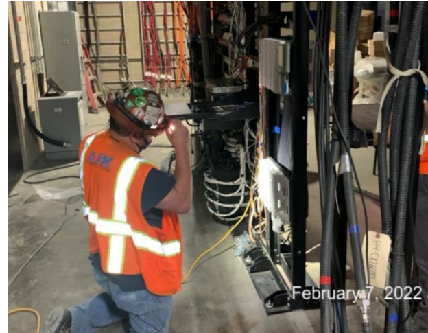
Communication rack installation at Grand Av/Arts District Station
