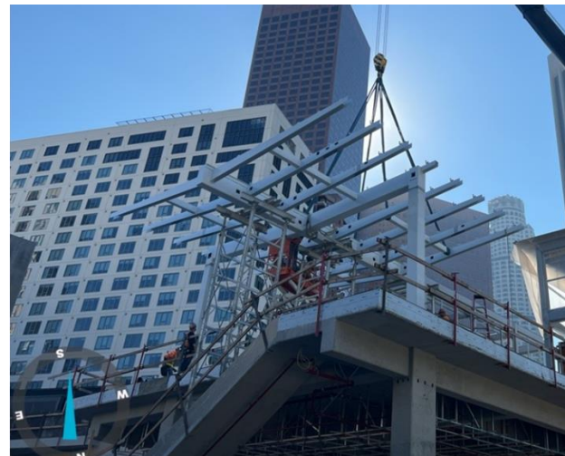
Canopy installation at Grand Av Arts/Bunker Hill Station
