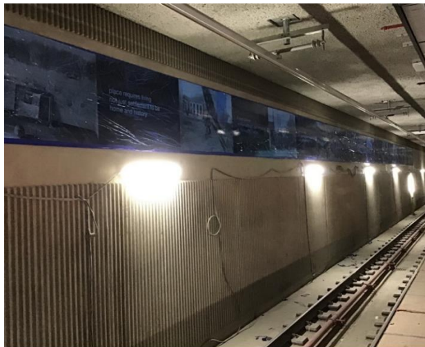
Porcelain enamel steel art panels at Platform Level at Historic Broadway Station
