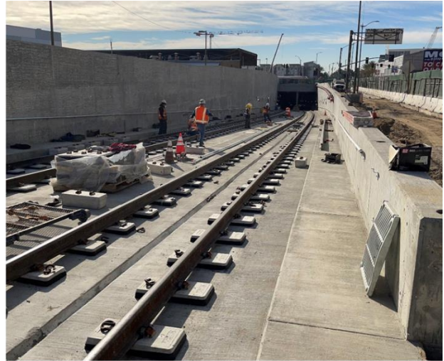
Trackwork on Alameda Leg
