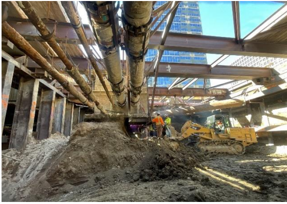
Station Entrance Excavation Activities in Century City
