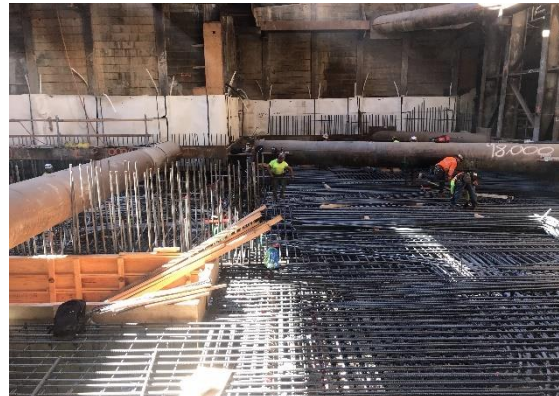
Rebar and Formwork for Wilshire/Rodeo Station Entrance
