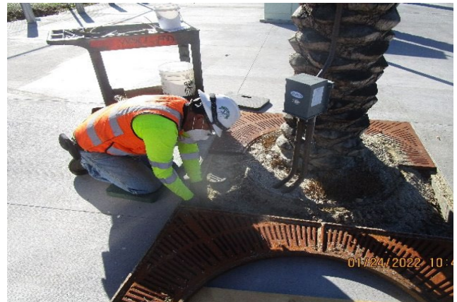
EXPO STATION - Bonding and grounding palm tree steel grates.
