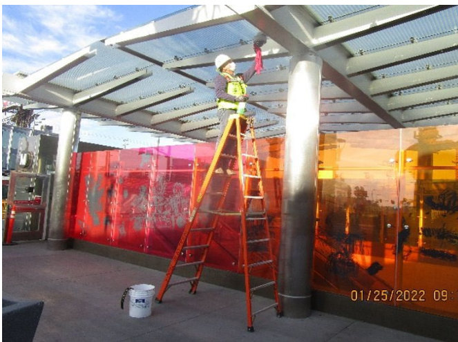
LEIMERT PARK STATION – Cleaned CCTV cameras throughout the main entrance plaza canopy.
