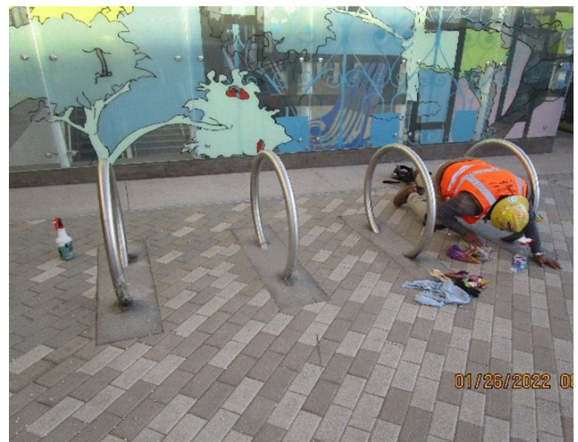
MLK STATION – Cleaning and polishing bicycle racks at the plaza.
