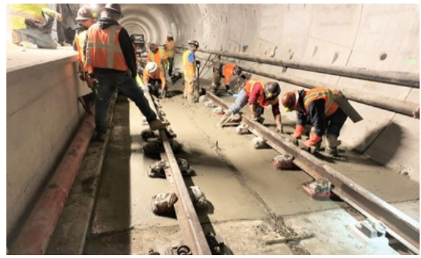
Track Installation in the Reach 1 Tunnel
