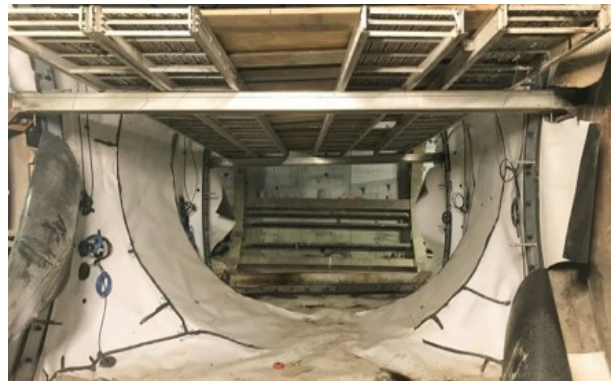
Cross Passage 21 (Reach 2) HDPE Installation
