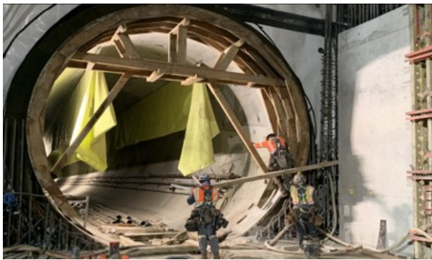
West End Wall at Wilshire/La Cienega Station
