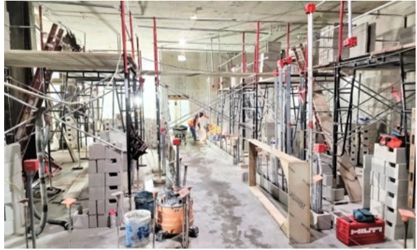
CMU Block Installation at Wilshire/Fairfax Station
