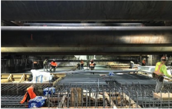
Concourse Rebar Installation at Wilshire/La Brea Station
