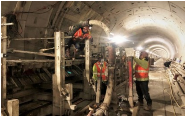
Walkway Concrete Placement in the Reach 1 Tunnel
