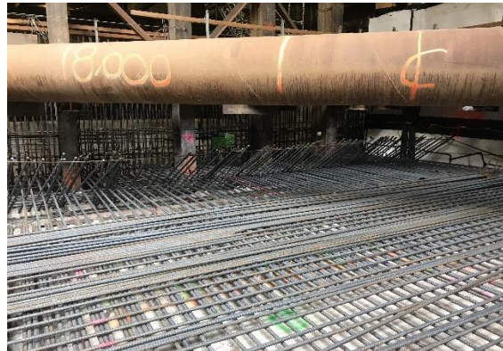
Rebar and Formwork for Wilshire/Rodeo Station Entrance
