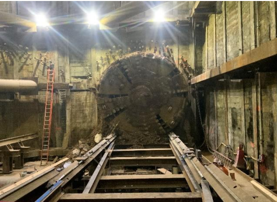
BR TBM Break-In at Wilshire/Rodeo Station
