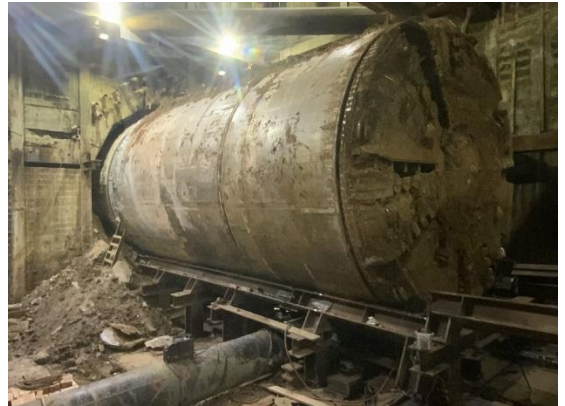
BR TBM Break-In at Wilshire/Rodeo Station
