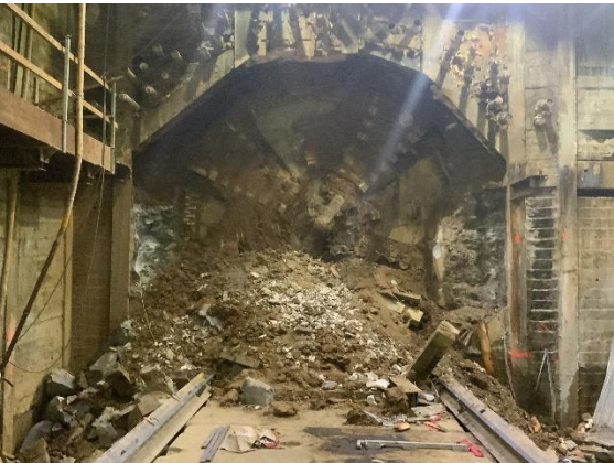
BL TBM Break-In at Wilshire/Rodeo Station
