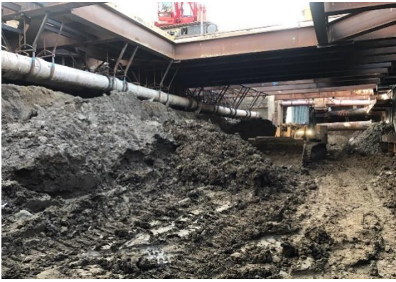
Station Entrance Excavation Activities in Century City
