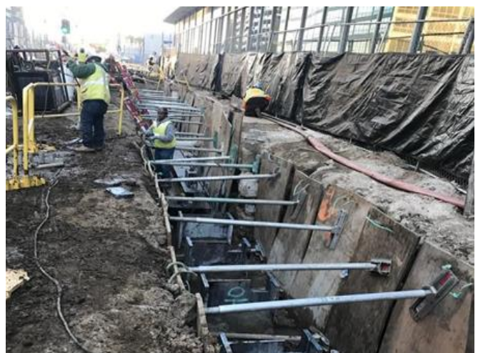
Support of Excavation Cap Beams at Westwood/UCLA Station
