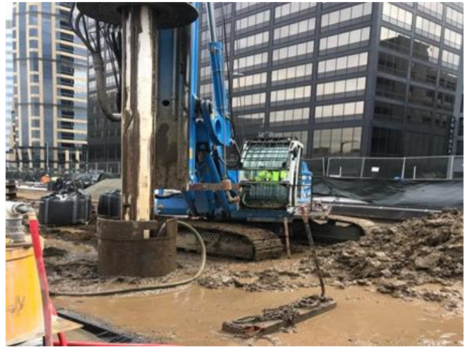
Dewatering Well Installation at Westwood/UCLA Station
