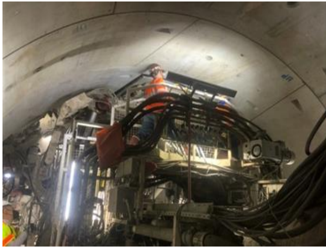
Ring Installation in the BR Tunnel
