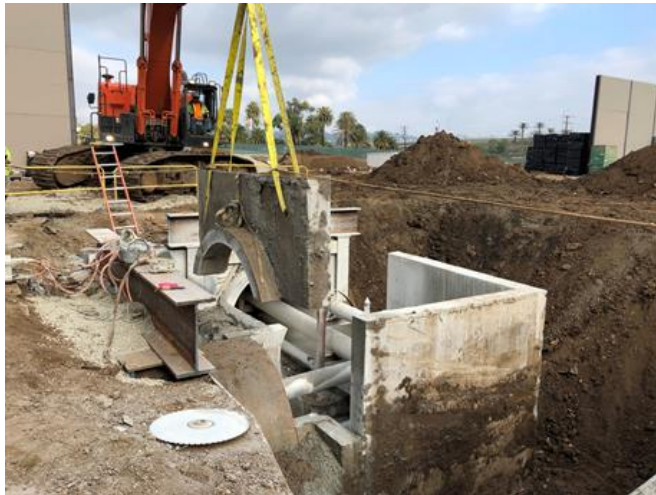
Vault 400 Wall Demolition for Steam Tunnel Relocation
