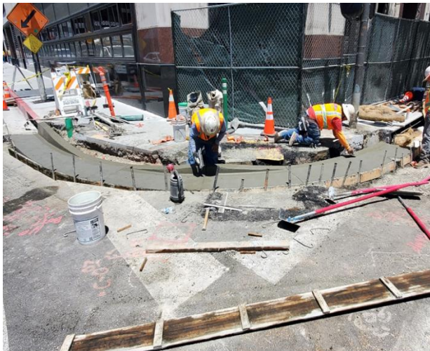
2nd & Spring Street curb and gutter concrete placement
