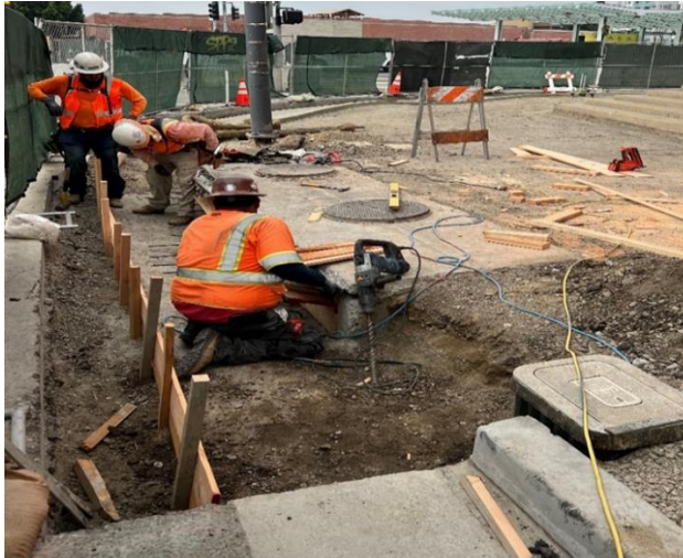
Curb and gutter at 1st Street corner
