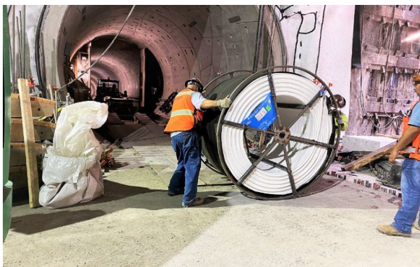
Reach 1 Tunnel Conduit Installation
