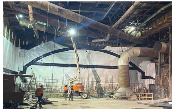
Level 2 Wall Construction at Wilshire/La Cienega
