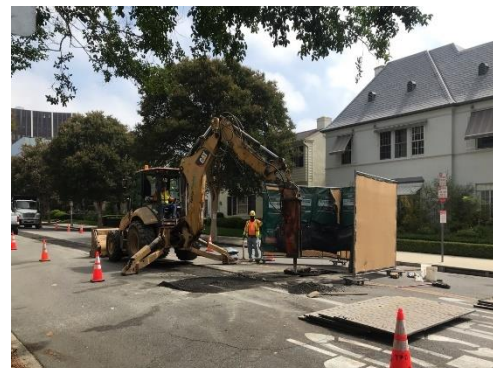
Cross Passage Dewatering Well Activities
