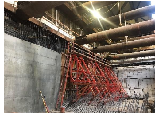
Wall Formwork at the Wilshire/Rodeo Station Entrance
