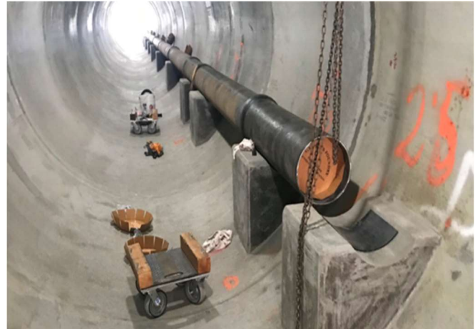
VA Steam Tunnel – Installation of 12-inch Ductile Pipe (Line B)
