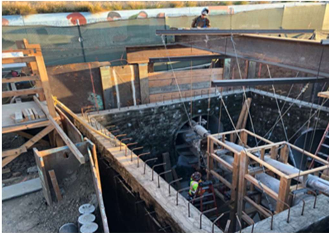
VA Steam Tunnel – Install temporary pipe supports in Vault 100
