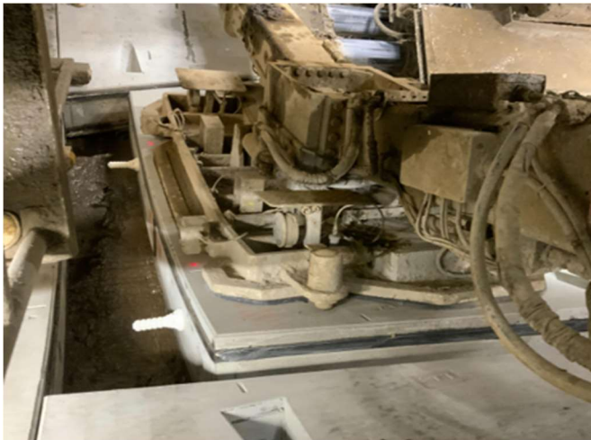
BR TBM – Segment Installation at Cross Passage 49
