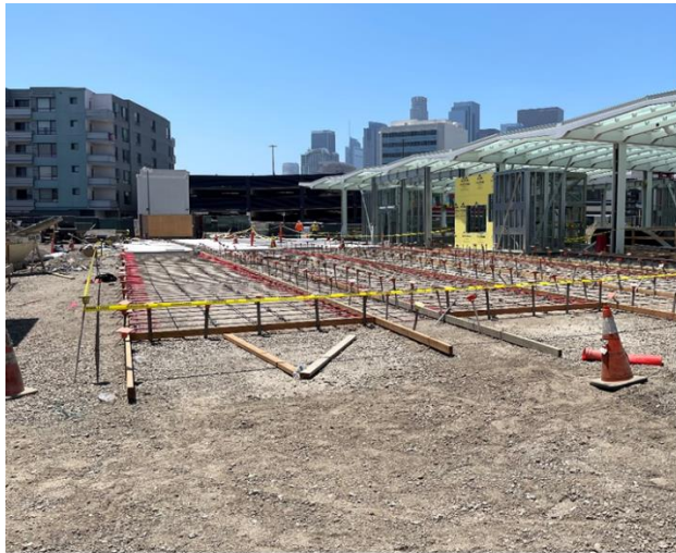
Plaza form and rebar for architectural paving at Little Tokyo/Arts District Station
