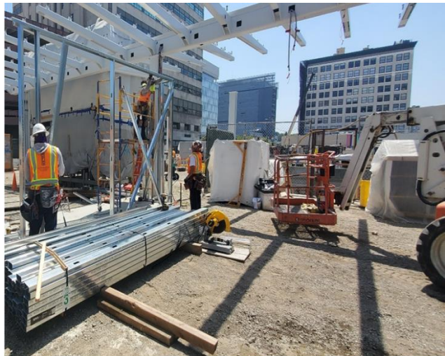
Installation of steel stud framing for plaza electrical closets at Historic Broadway Station
