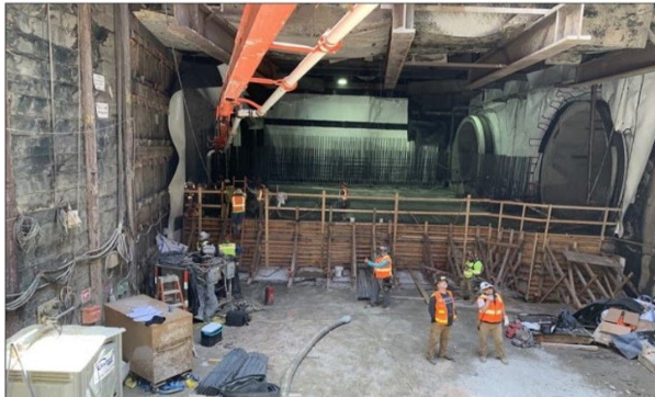
Concrete Invert Placement at Wilshire/Western Shaft
