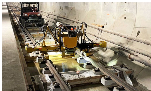
Reach 1 (South) Track Installation
