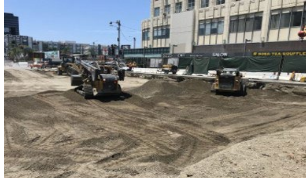
Wilshire Boulevard Restoration at Wilshire/La Brea Station
