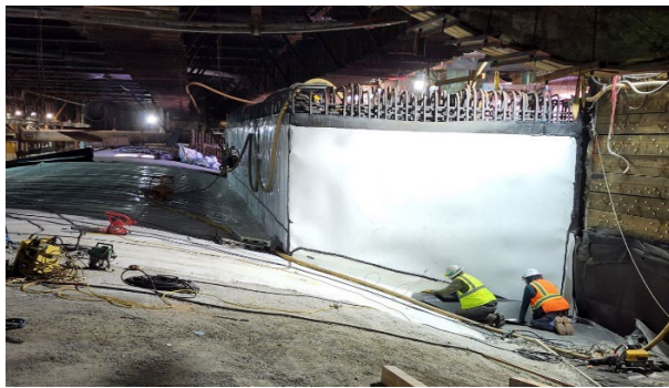
Above Roof Construction at Wilshire/Fairfax Station
