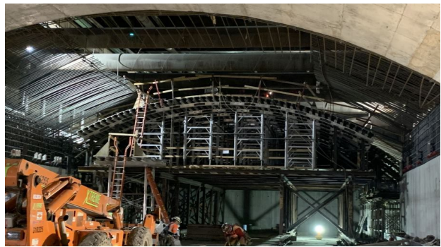
Roof Construction at Wilshire/La Cienega
