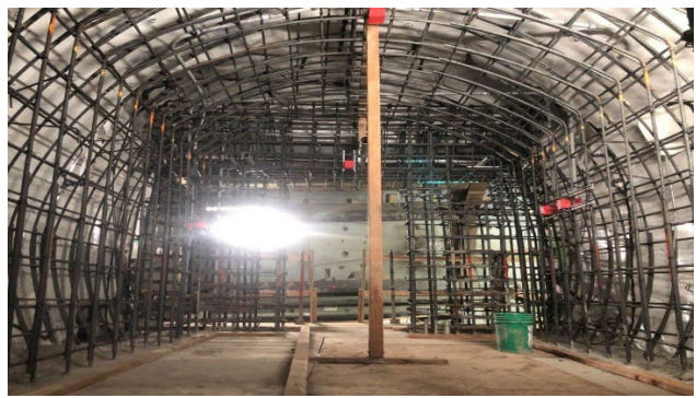
Cross Passage 23 Construction (Reach 3)
