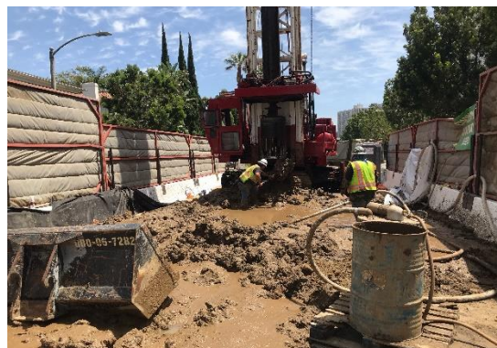
Cross Passage Dewatering Well Activities
