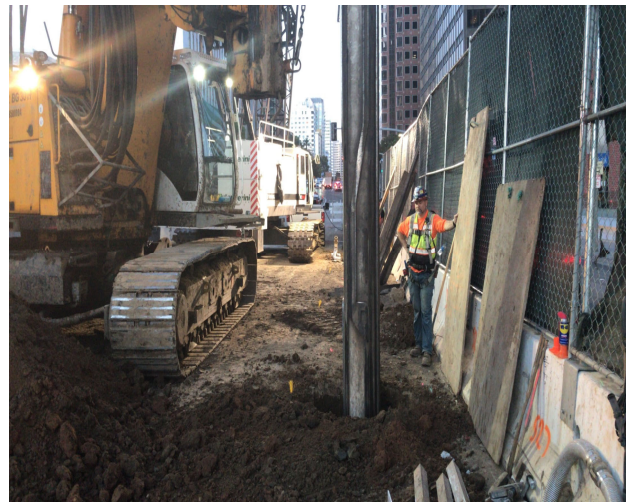
Westwood/UCLA Station SOE Pile Drilling Wilshire Blvd. Median
