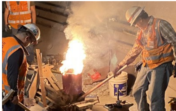
Rail Welding in the Reach 1 Tunnel
