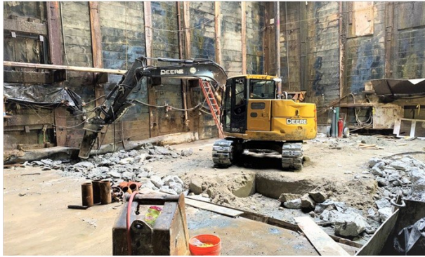
Temporary Slab Removal at Wilshire/Western Shaft
