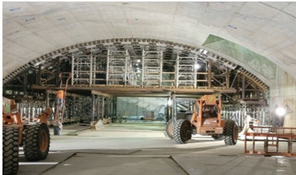
Roof Formwork Installation at Wilshire/Fairfax Station
