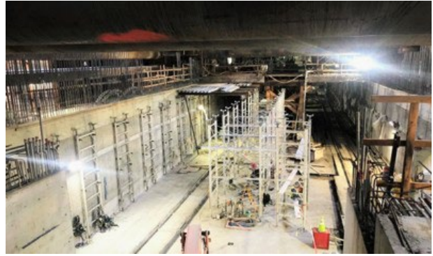
Concourse Shoring at Wilshire/La Brea Station
