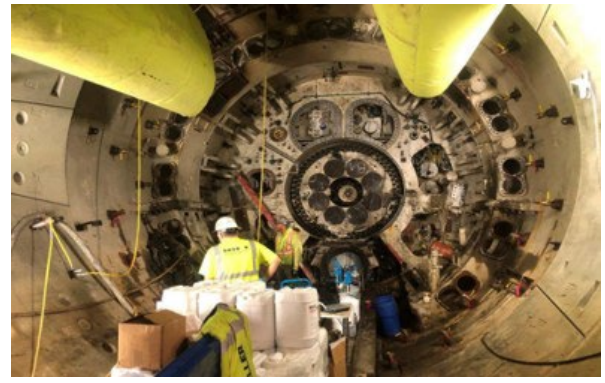
Cutterhead Grouting at South (Red) TBM (Tail Track)
