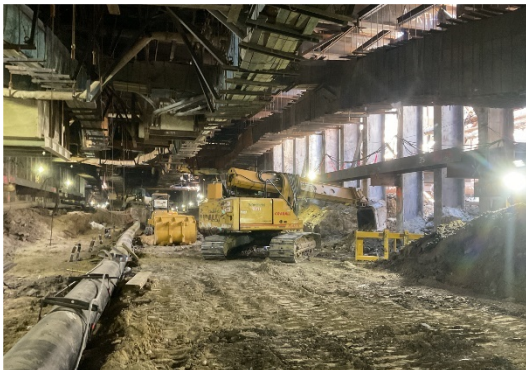
Excavation and Utility Support Activities West of the Launch Box in Century City
