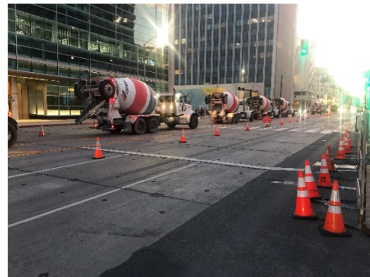
Preparations for Concrete Placement at Wilshire/Rodeo Station Entrance for Invert Slab
