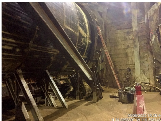
BR TBM Relaunch at Wilshire/Rodeo Station
