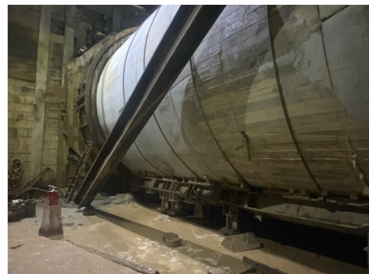
BL TBM Relaunch at Wilshire/Rodeo Station
