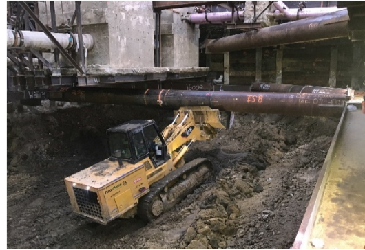
First Level Strut Installation Activities for Station Entrance in Century City
