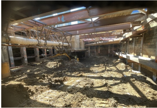
Station Entrance Excavation Activities for Station Entrance in Century City
