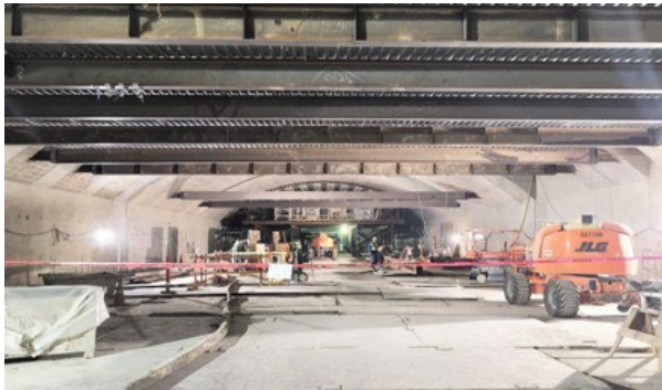
Plenum Construction at Wilshire/Fairfax Station
