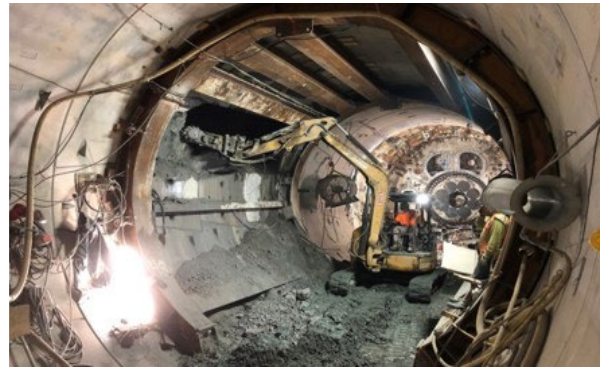
Cross Passage 26 Excavation (Reach 4)
