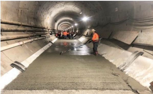
Reach 2 (North) Invert Concrete Placement
