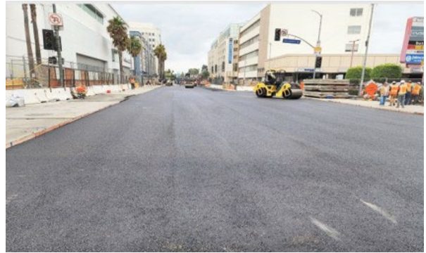
Wilshire Boulevard Restoration at Wilshire/La Brea Station
