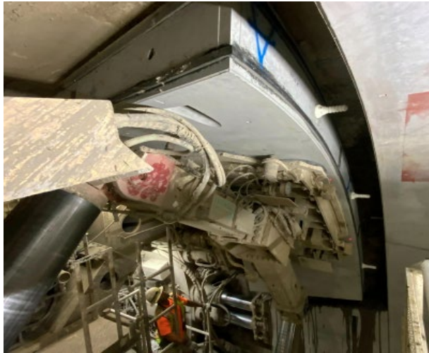
BL Tunnel - Ring Erection (Ring 1069)
