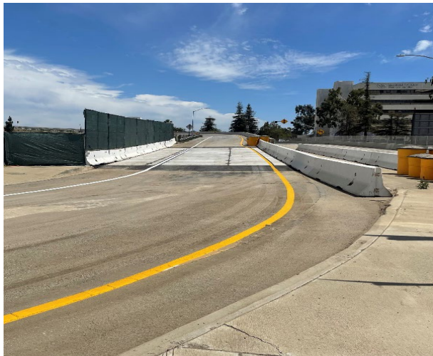
Westwood/VA Station Temporary Decking Installation at I-405 On/Off Ramps
