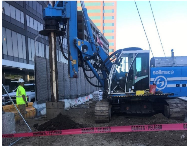
Westwood/UCLA Station Dewatering Well Installation (DW 29)
