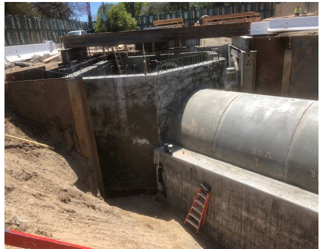
Westwood/VA Station Concrete Wall Placed for VA Steam Line Vault 400
