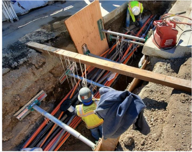
Excavation for AT&T vault along Spring St.
